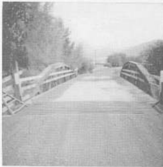
23C571 Morgan Bridge
