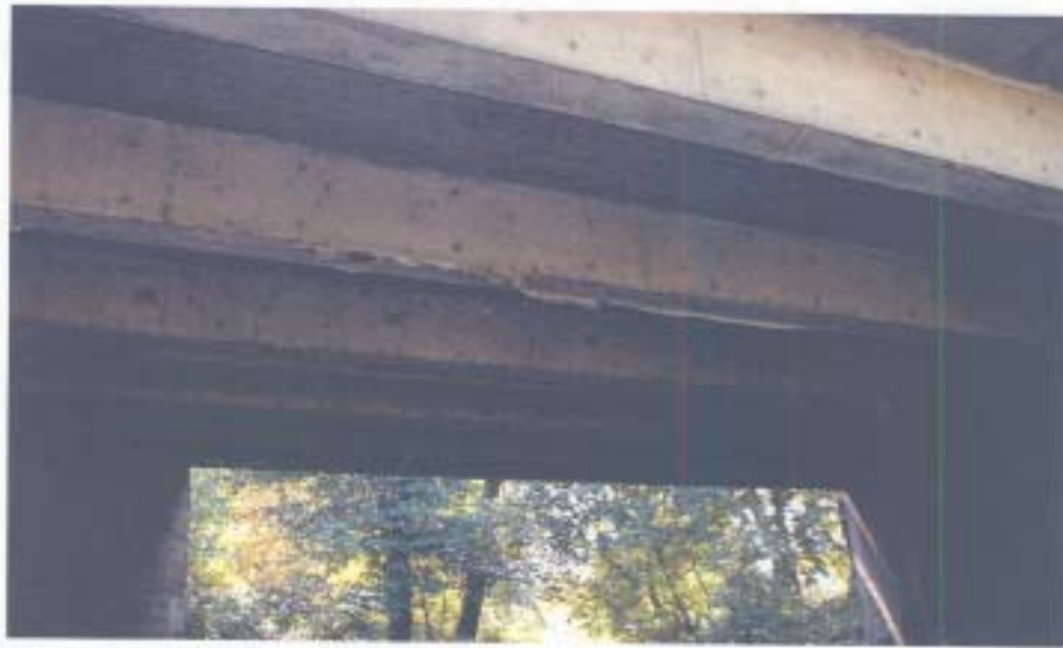
Photograph No. 5 — Superstructure.
