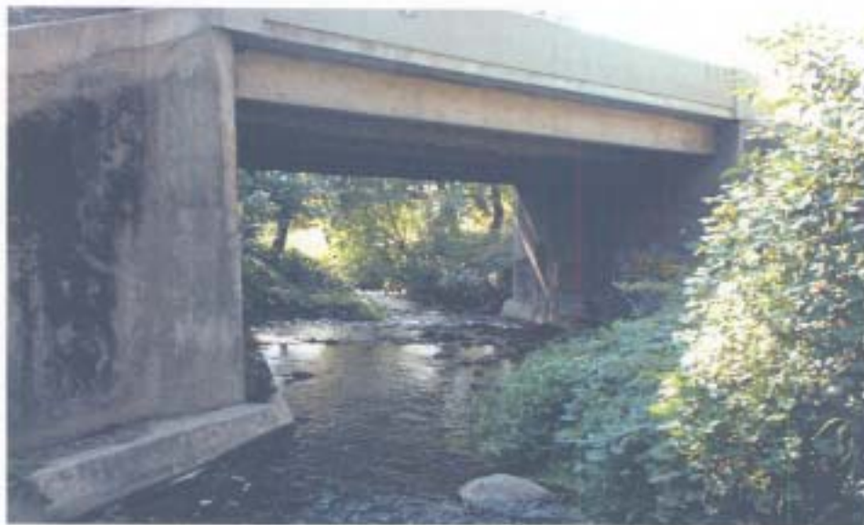
Photograph No. 4 — Elevation looking south.
