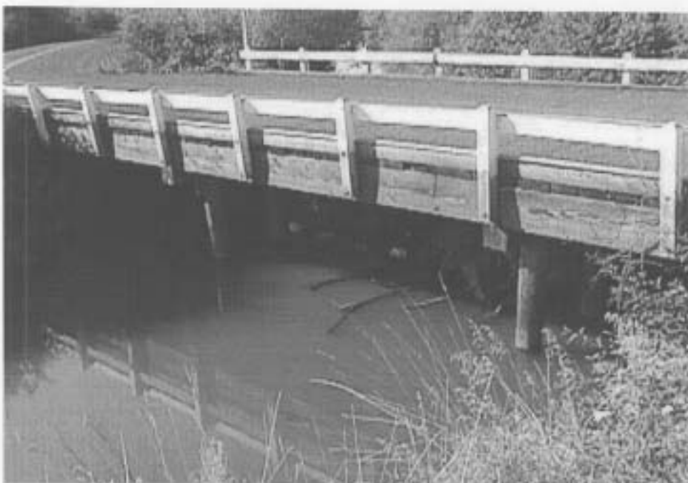
Elevation Viewing West
