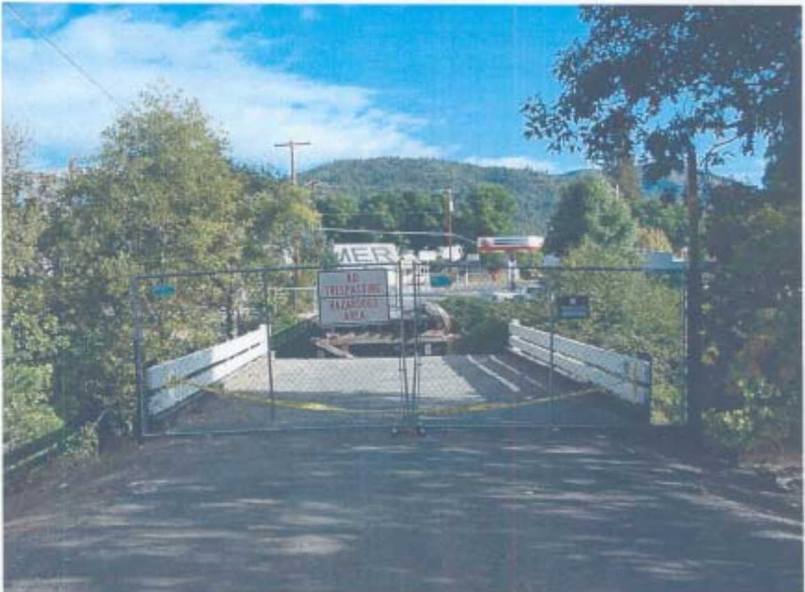
Bridge 29C211 - South Approach
