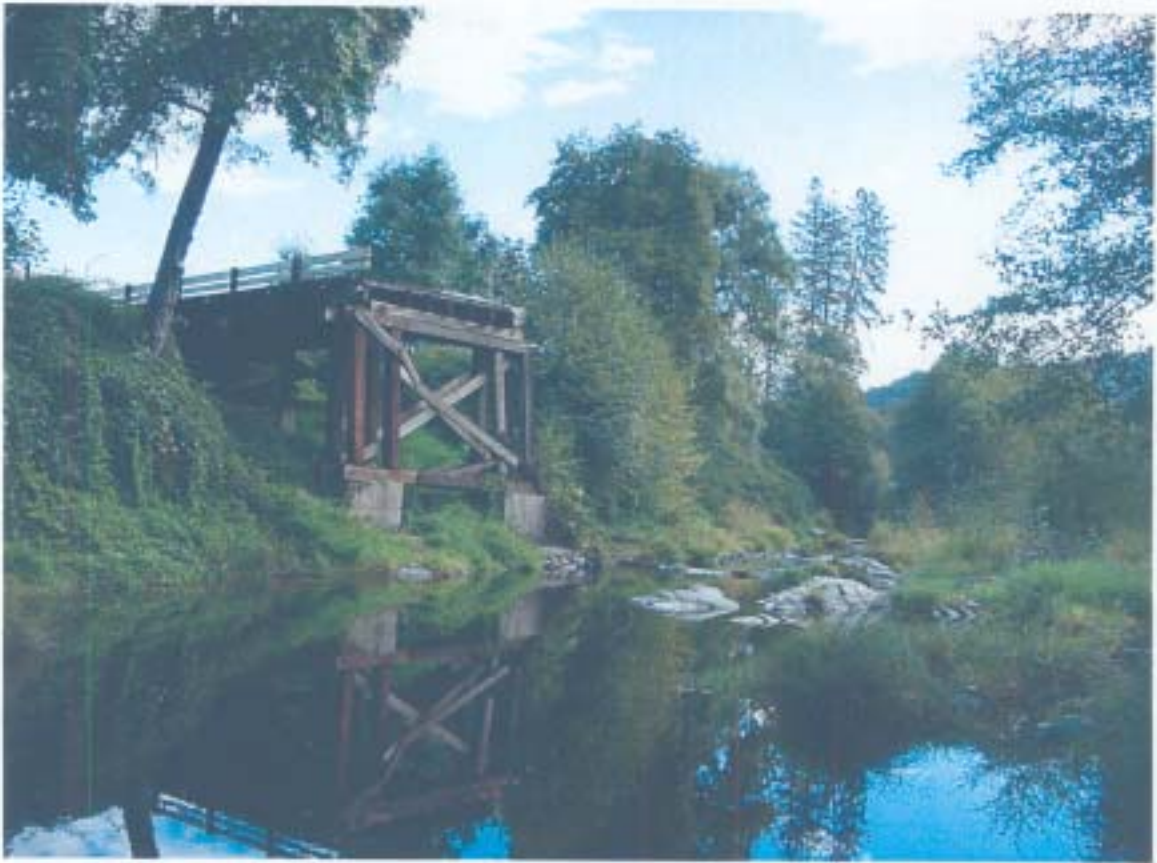
Bridge 29C211 - Downstream
