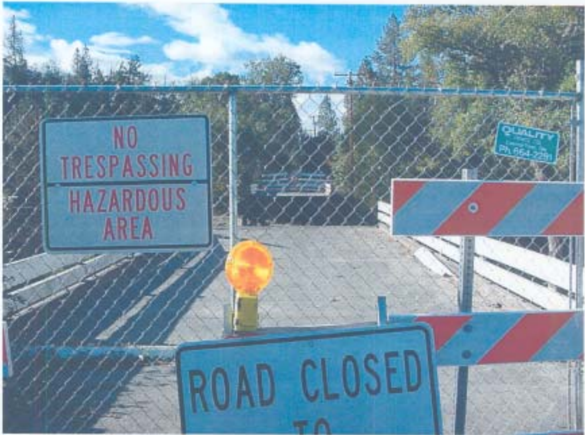
Bridge 29C211 - North Approach
