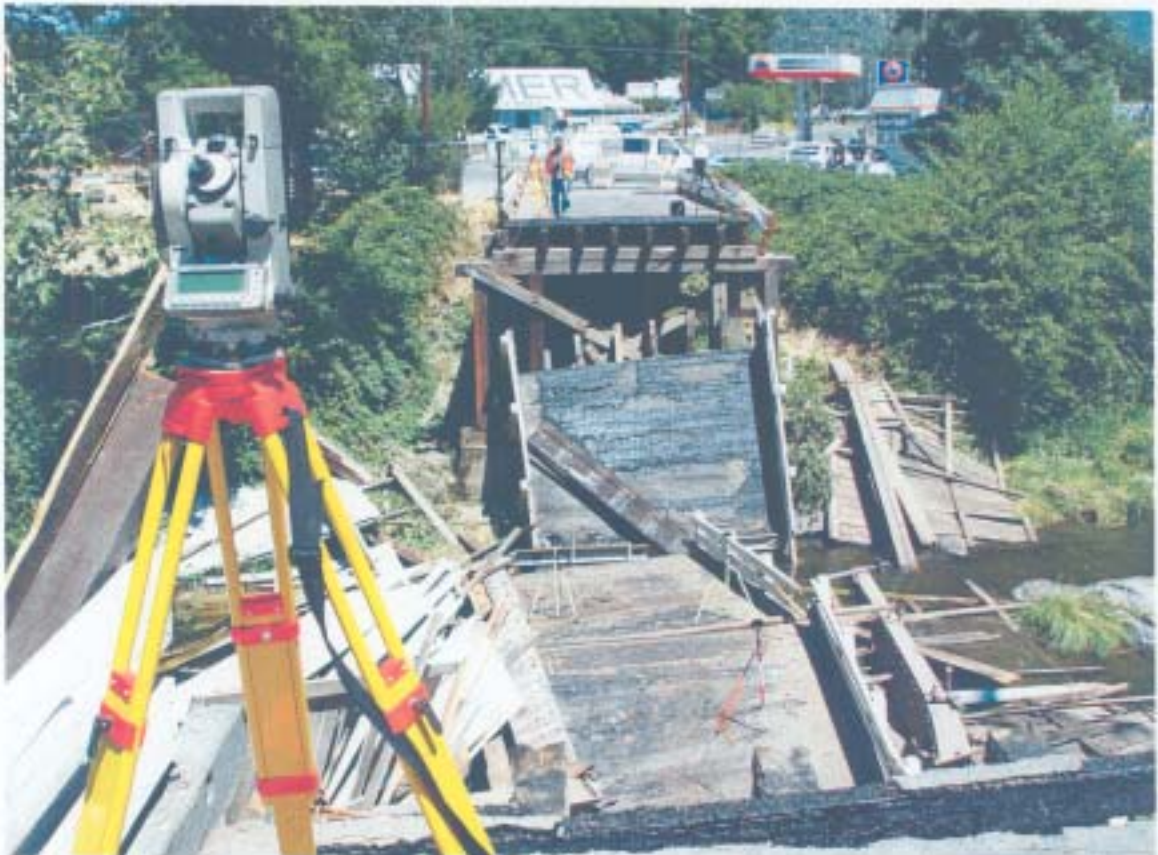
Bridge 29C211 - In-stream
