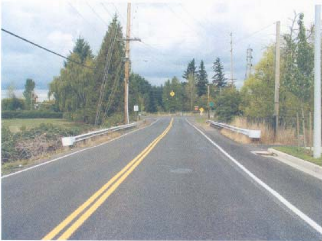
SE 190 th facing north over Johnson Creek
