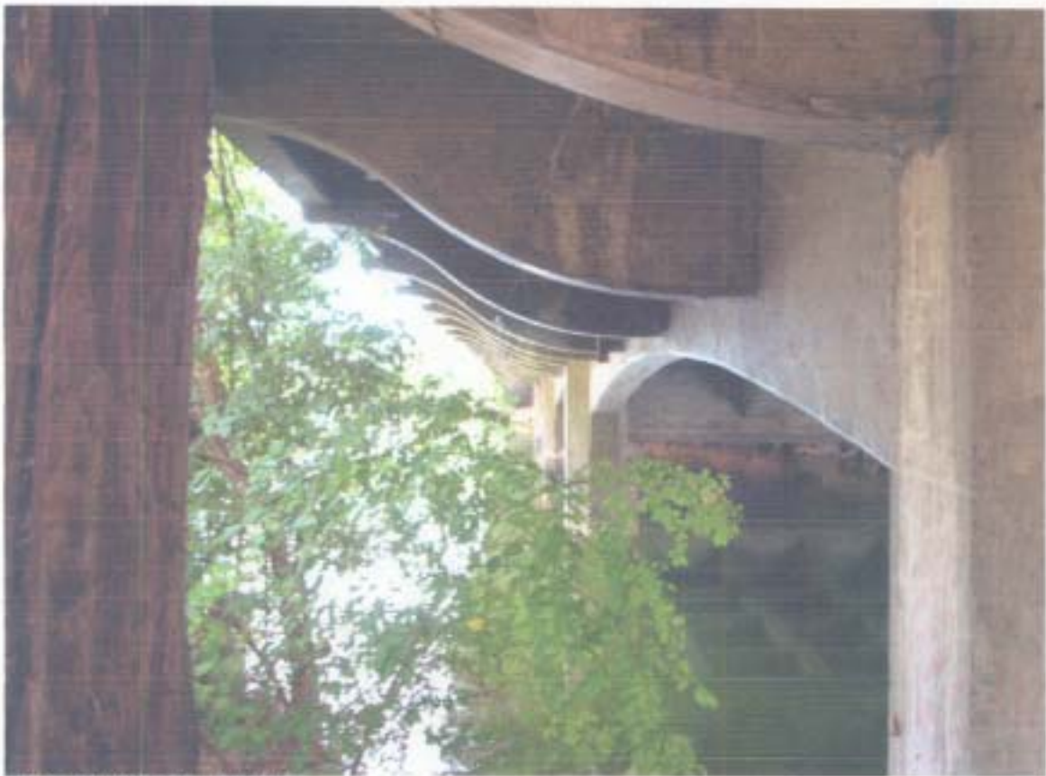
Underside of bridge overhang.
