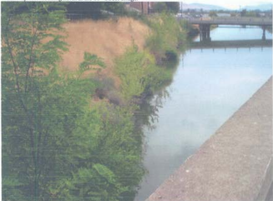
Waterway looking south from the 11 th Street bridge.
