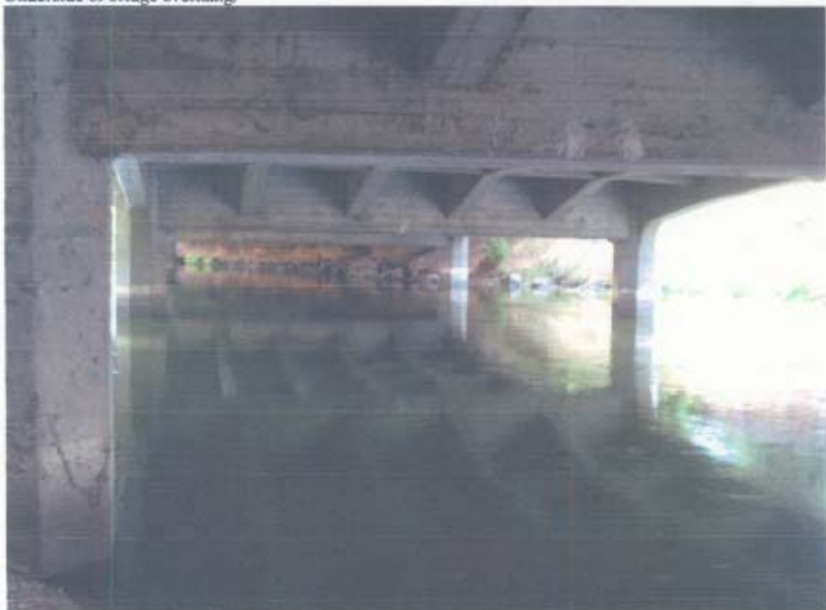
Numerous bridge columns in the active flowing stream.
