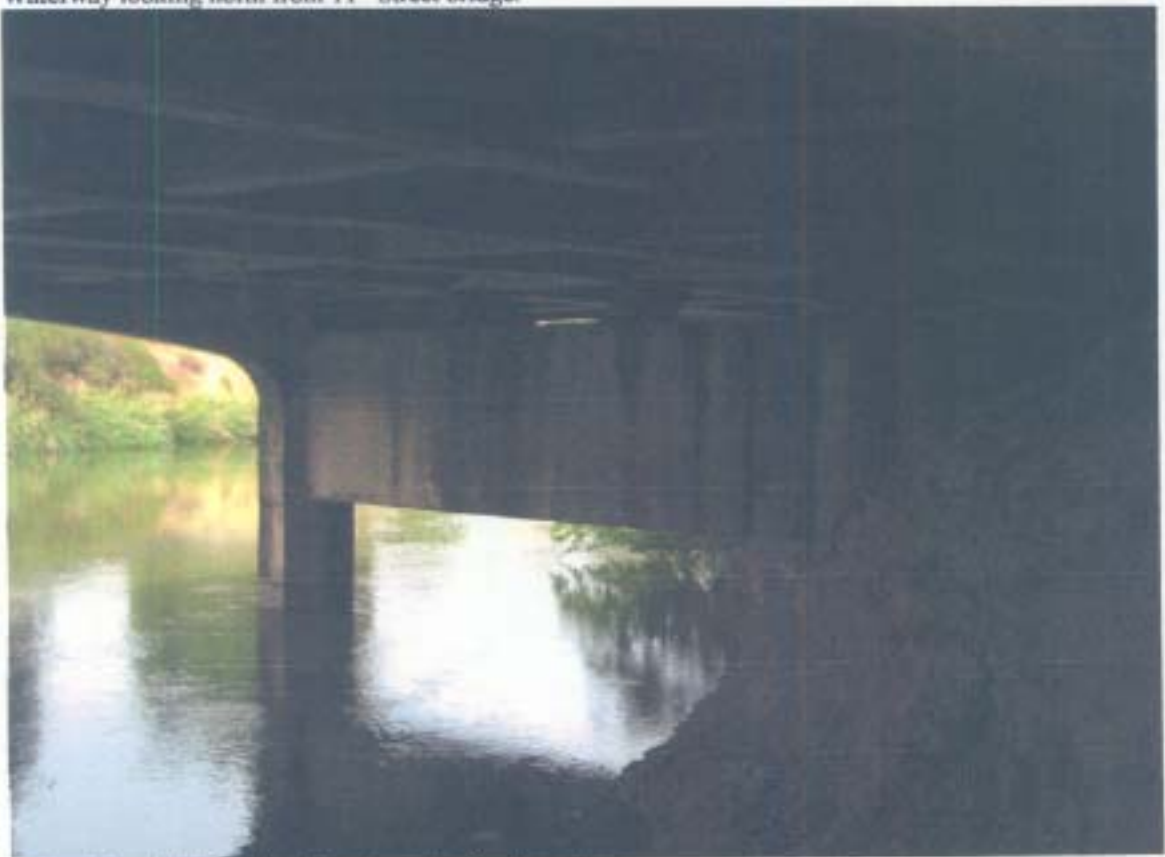
Underside of bridge with column in active flowing stream.
