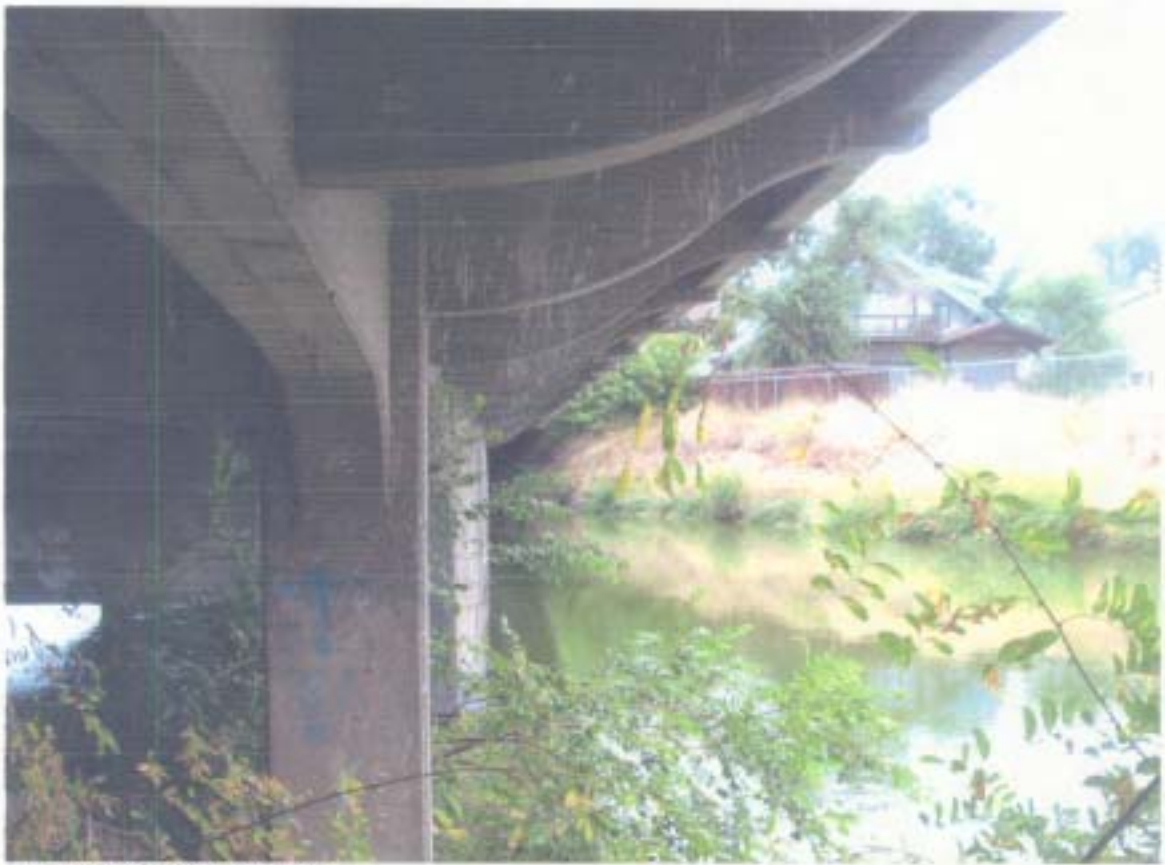
Underside of bridge overhang.
