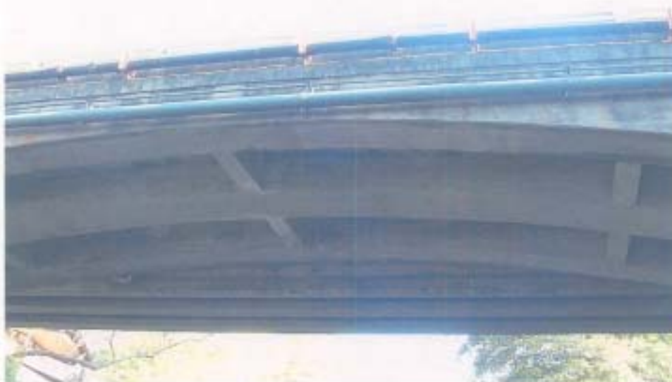
Photograph No. 2 — Superstructure.
