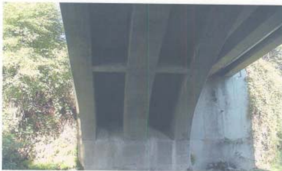
Photograph No. 3— Superstructure.
