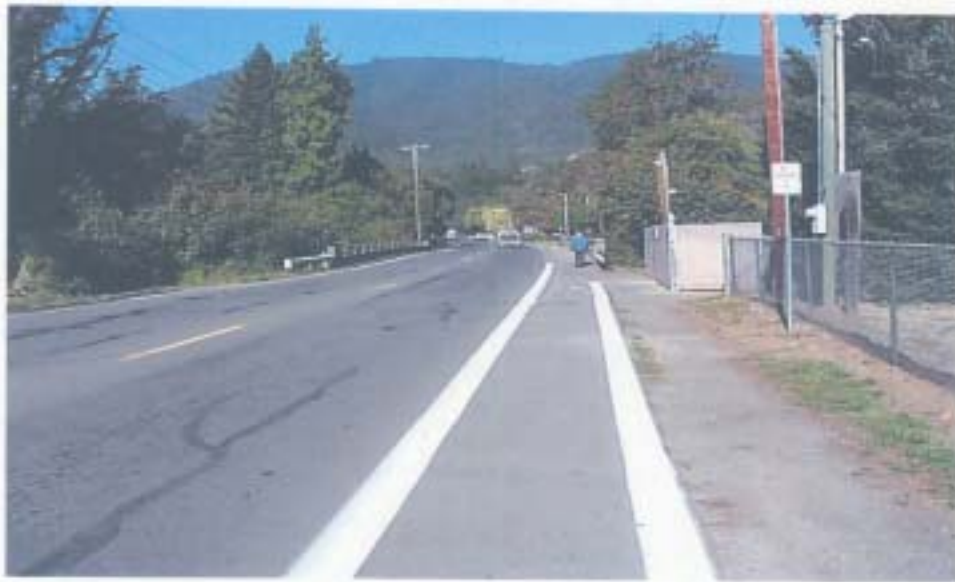
Photograph No. 7— Approach looking west.
