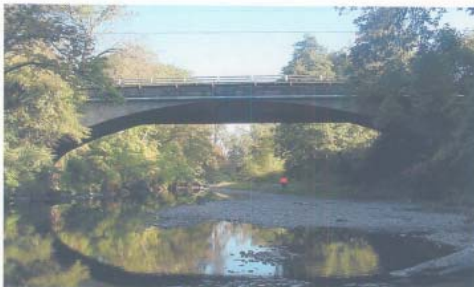
Photograph No. 1 — Elevation looking north.
