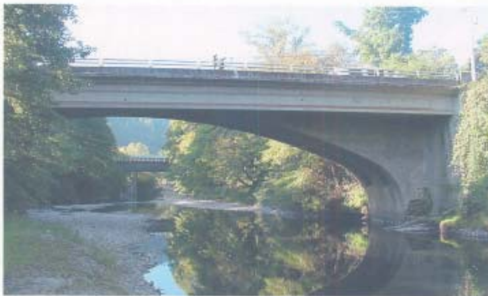
Photograph No. 4— Elevation looking south.
