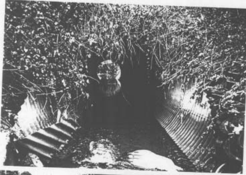
Looking through culvert from upstream end.
