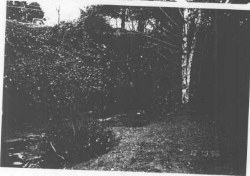
Looking at upstream end.
