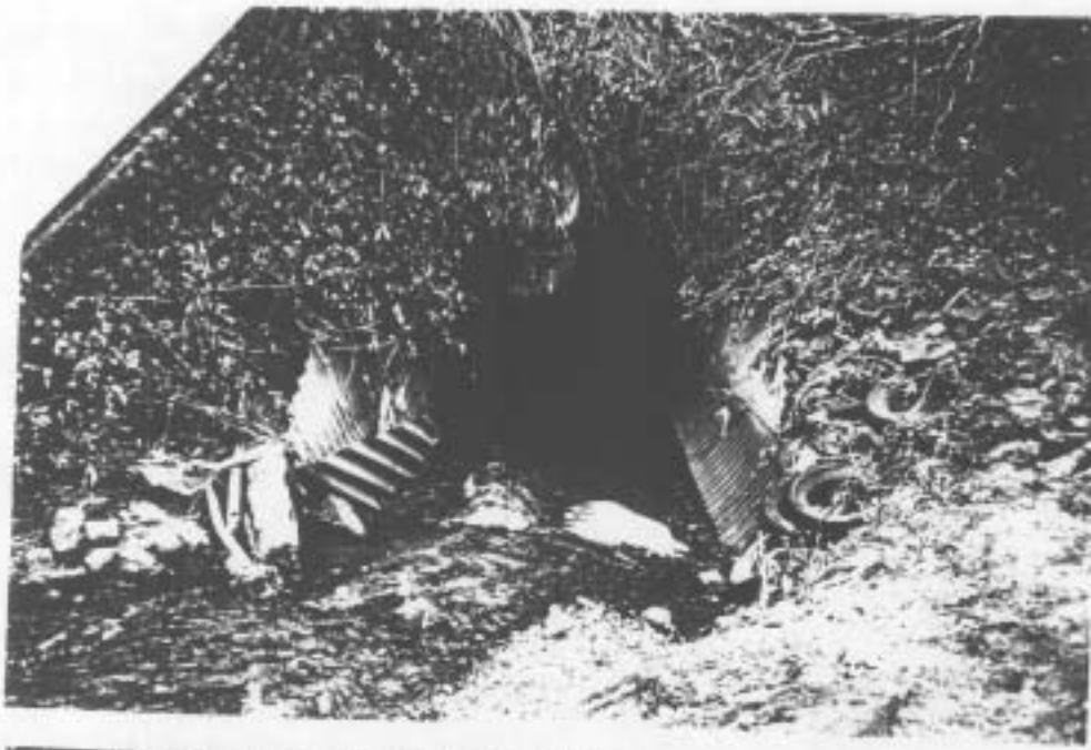
Looking at upstream end.
