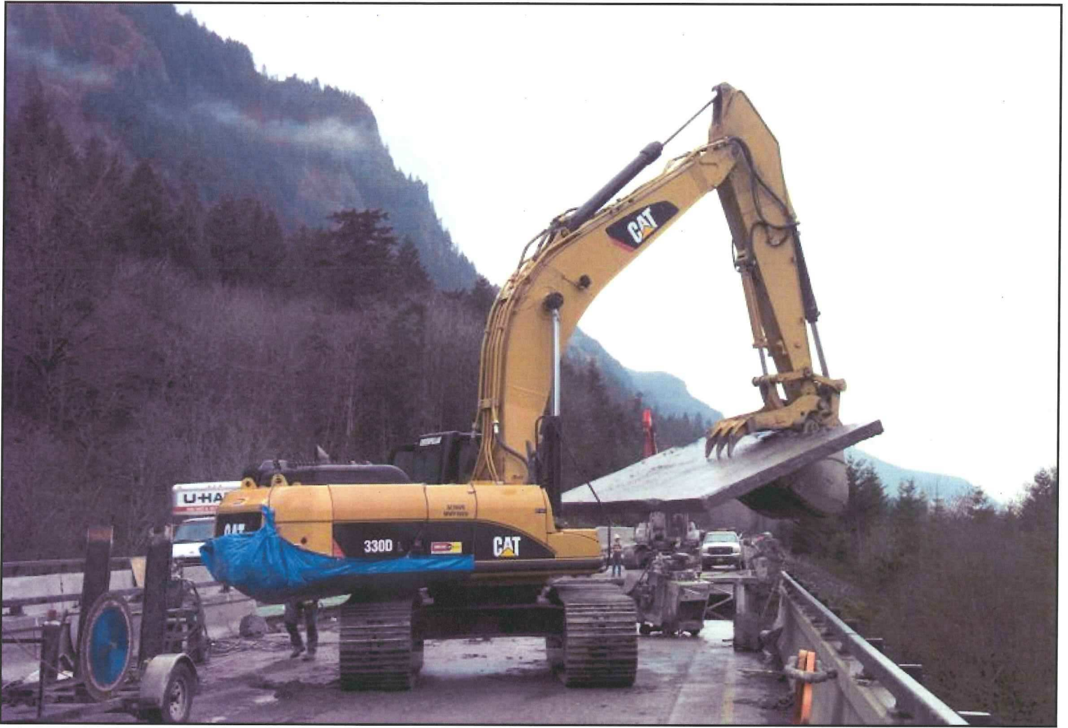
I-84: Dodson – Tanner Creek, Bundle 209: Demolition started in winter of 2009.
