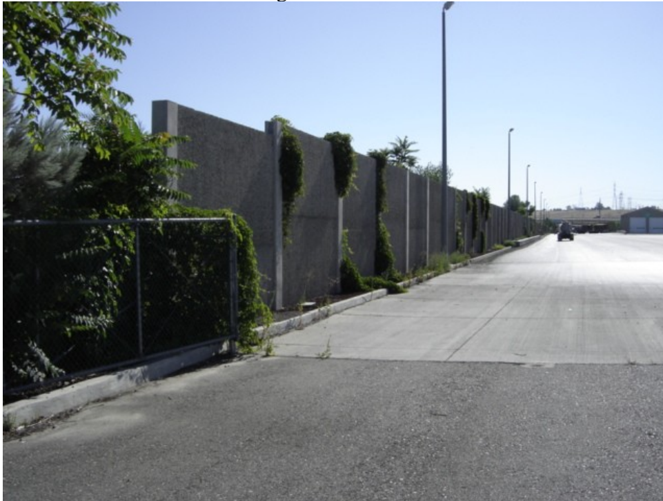
Picture #1. Sound Wall looking East.
