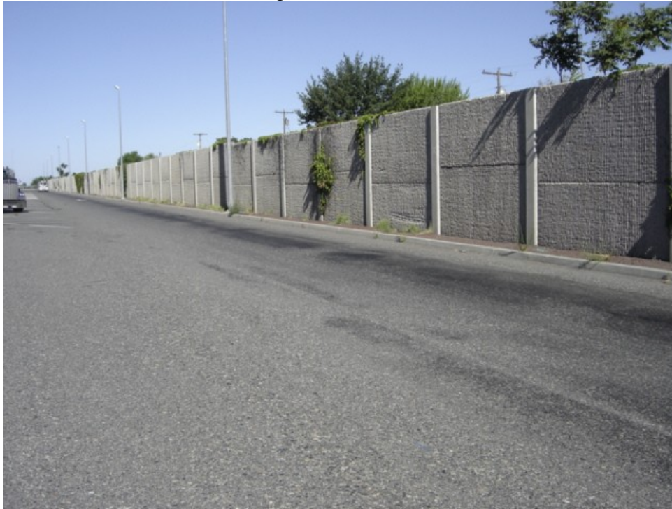
Picture #3. Sound wall looking West.
