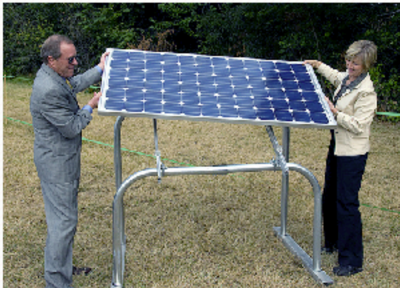
Gov. Ted Kulongoski and Portland General Electric CEO Peggy Fowler install the first solar panel last month. Picture courtesy of OregonDOT
