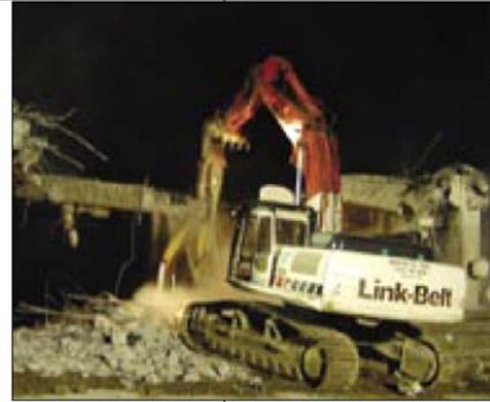
An excavator helps demolish an old bridge.
