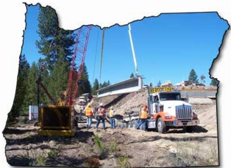
Highway 4 over Crescent Connection
