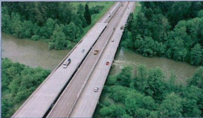
The Coast Fork Willamette River Bridge on Interstate 5 near Creswell is an OTIA III State Bridge Delivery Program replacement bridge with bioswales and specialized inlets that help remove stormwater pollutants.
