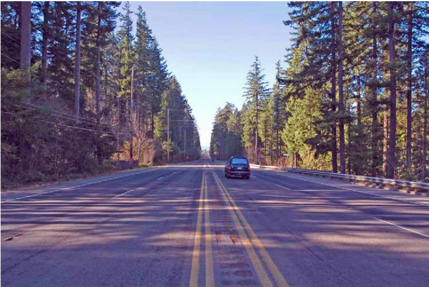
View To The West Of The Existing Condition In The Corridor --- near E. Wildwood Avenue
