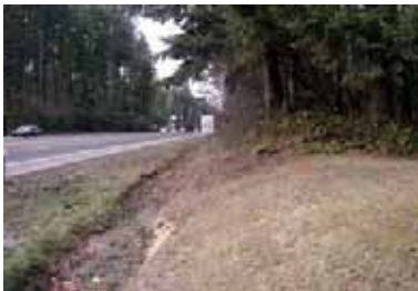
View to the west of US 26.
