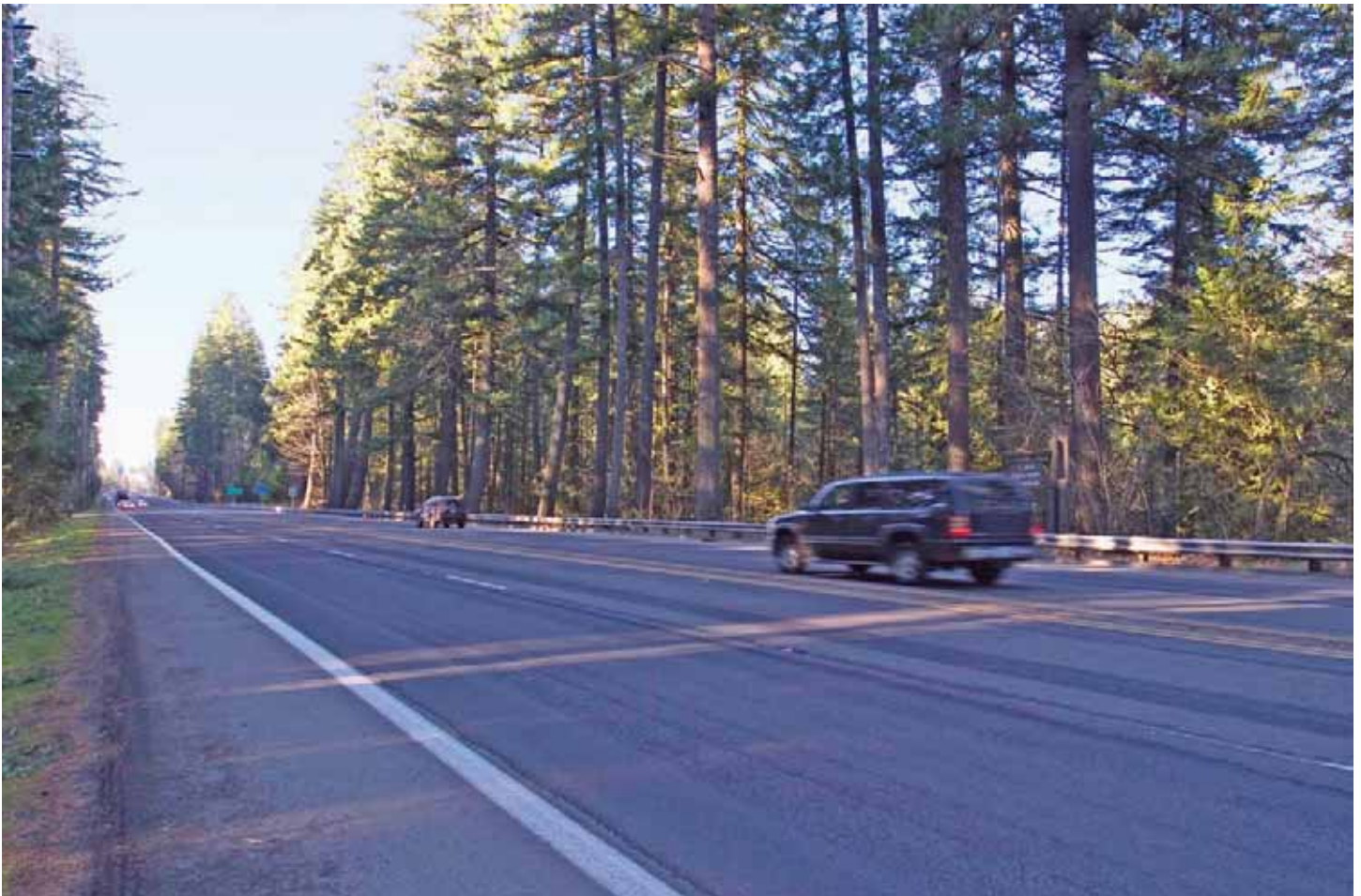
The Existing Condition In The Corridor --- Dwyer Area, View To The West
