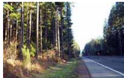
View to the east of the northern shoulder of US 26.
