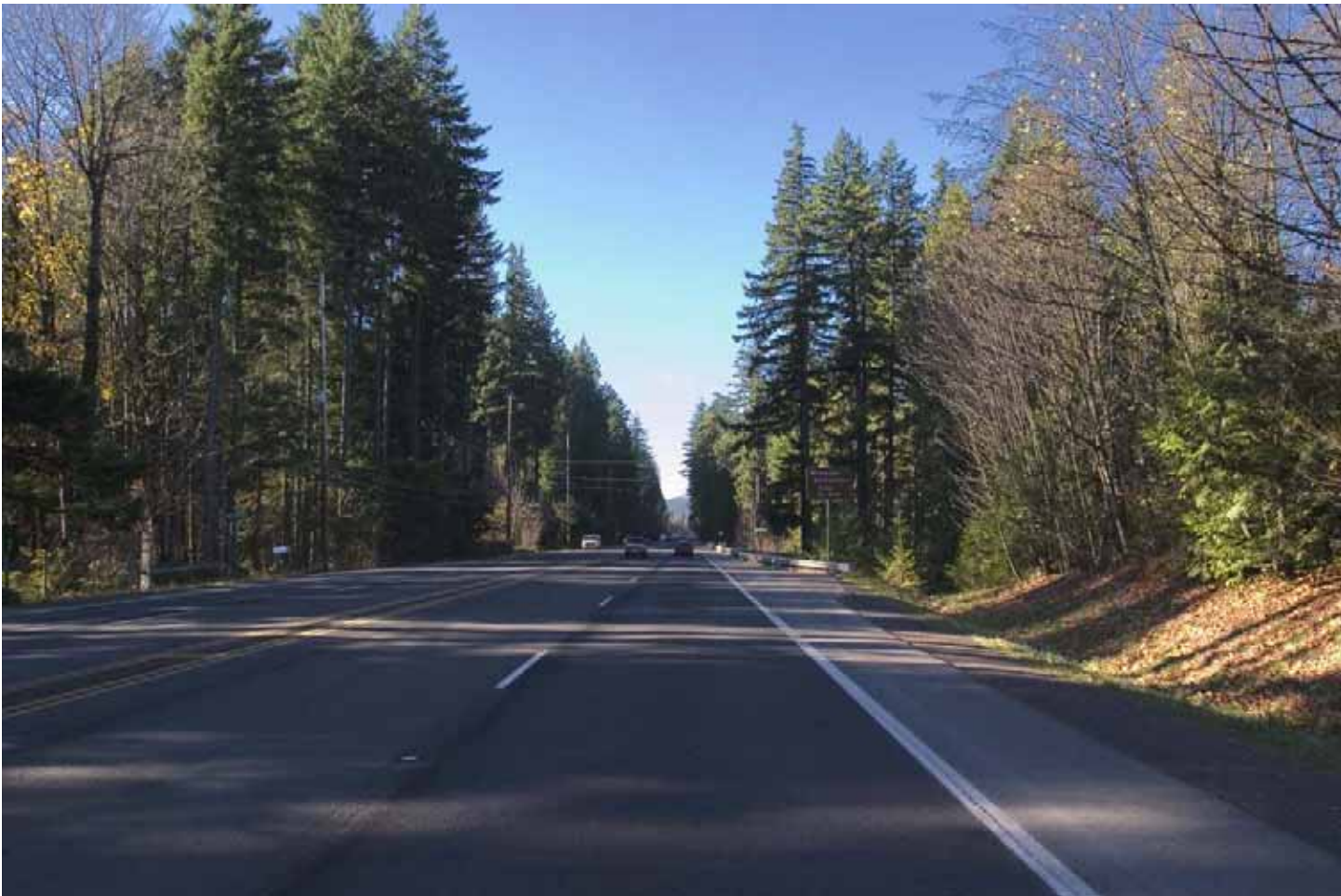
View To The West Showing The Existing Condition In The Corridor
