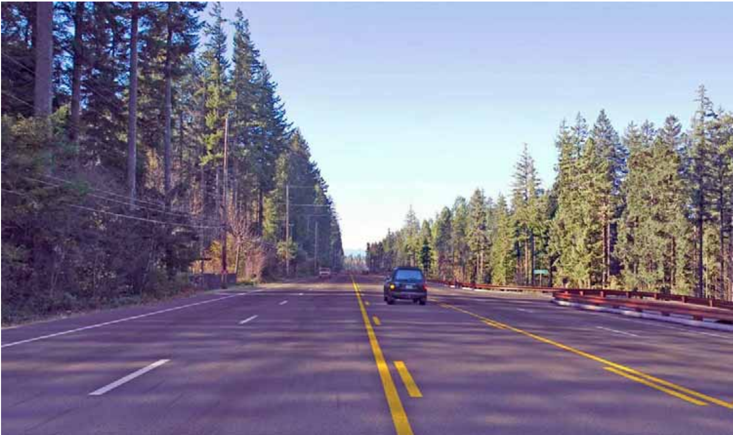
Illustrative View Simulating The Widen to the North Alternative --- near E. Wildwood Avenue
