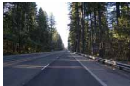
View to the west, in the Dwyer Area.
