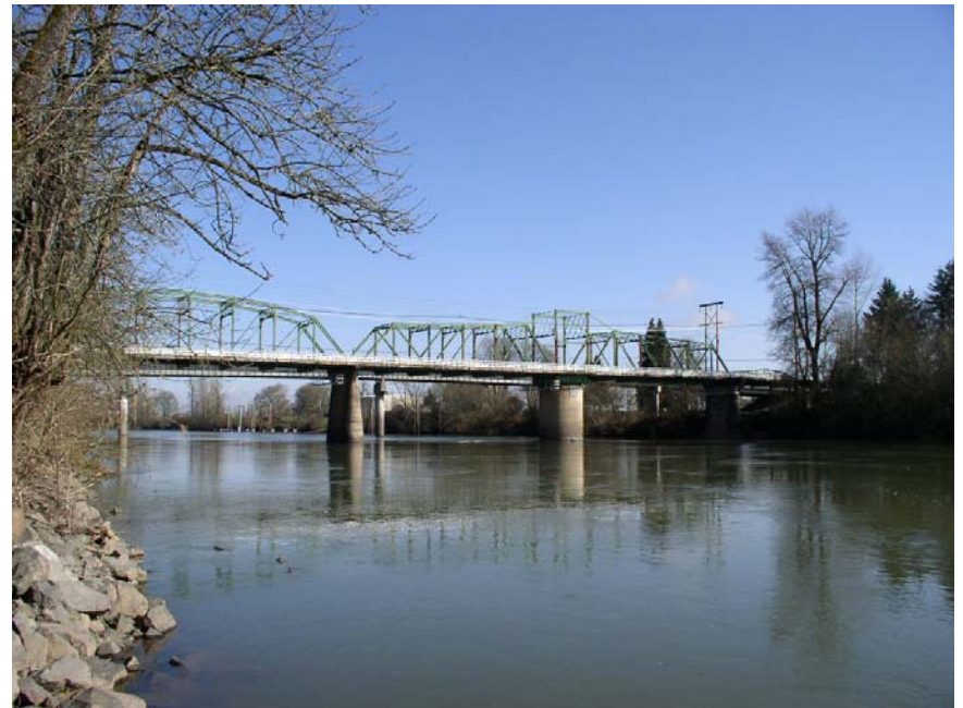
Van Buren Bridge, contemporary view to north.
