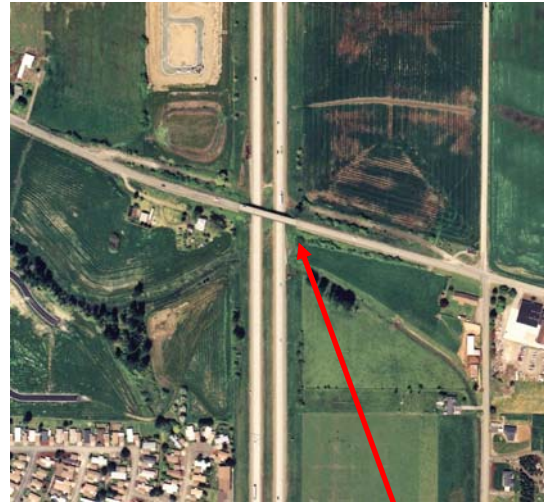
Grand Prairie Road Bridge (one out of four bridges being improved)
