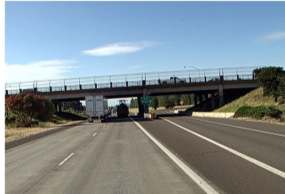
View of I-5 Northbound and Santiam Hwy Overpass
