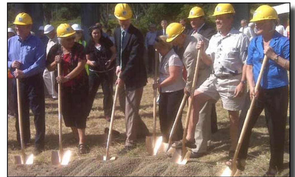
Federal, state and local officials break ground for the I-5 Willamette River Bridge replacement.
