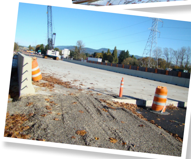
Canoe Canal Bridge ready for final lane paving early in 2011.
