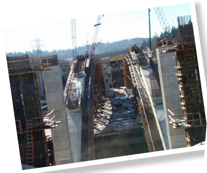
Arch ribs formed for the new Willamette River Bridge.
