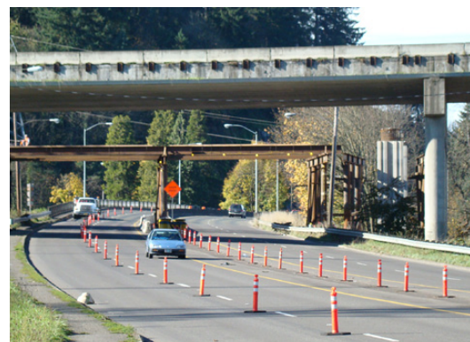
Bridge falsework spans Franklin Boulevard.
