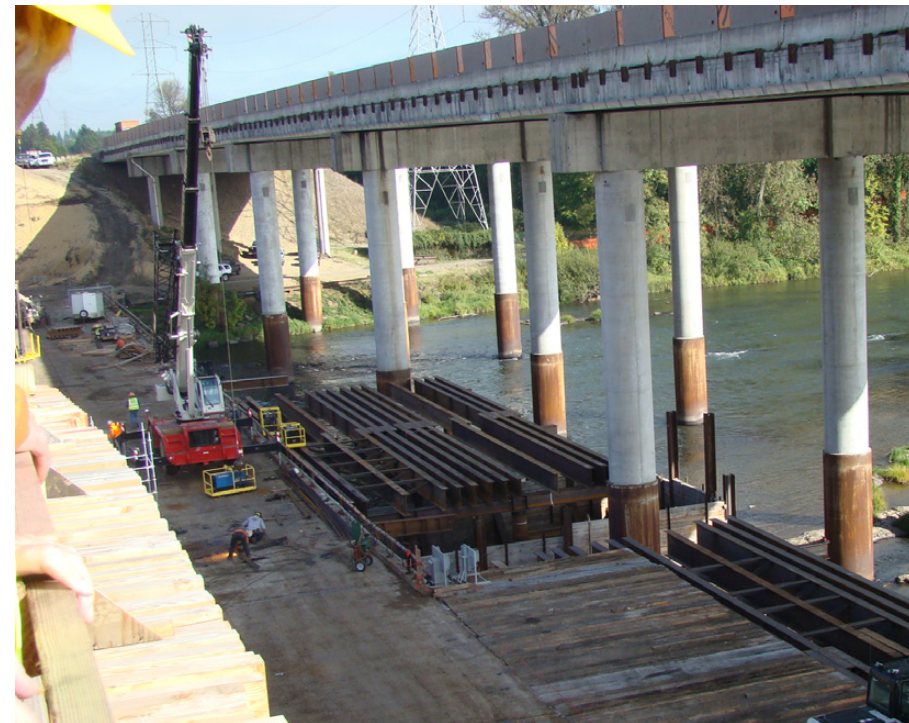
Building a new work bridge east of the existing bridge.
