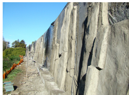
Sculptured concrete work on sound wall for Laurel Hill Valley neighborhood.
