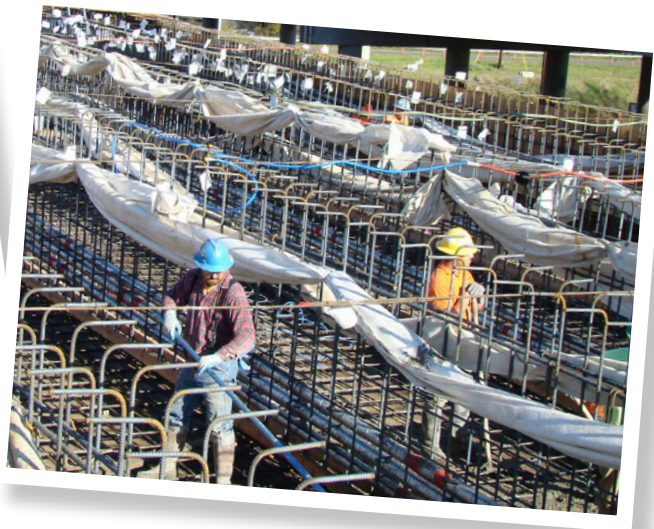
Box girder beams being poured over I-5 northbound off-ramp.
