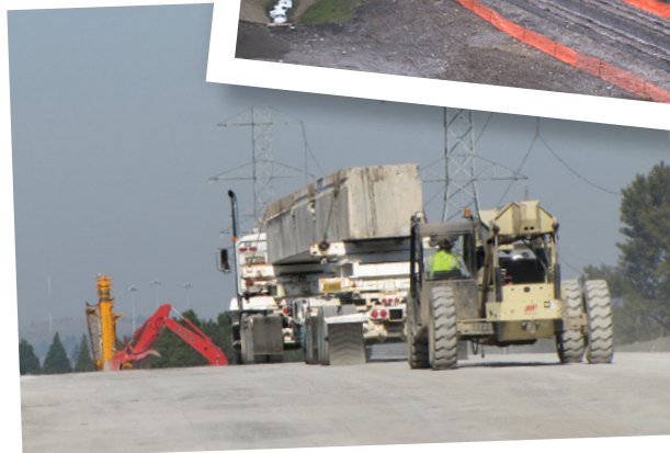
Each bridge beam is so large, it takes its own truck.
