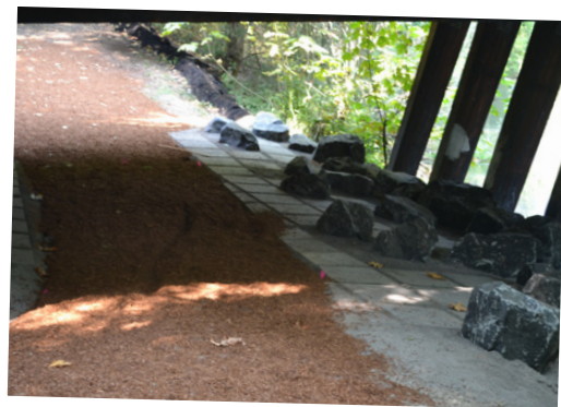
Trail enhancements under the Walnut Road bridge in Whilamut Natural Area.
