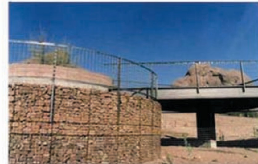
GABION WALL WITH RAIL
