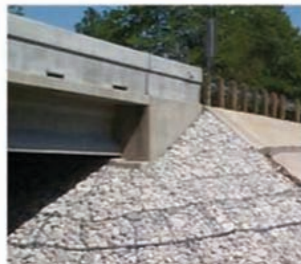
GABION END BENT
