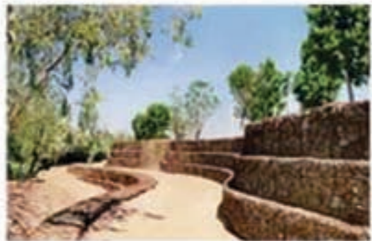
GABIION TERRACED WALLS
