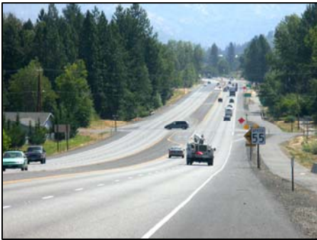
Shoulders and median on Highway 199 in the west segment; lack of safe left turn areas.
