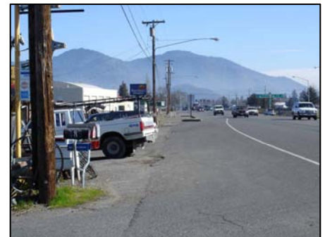
Unrestricted access on Highway 199 near Tussey Lane
