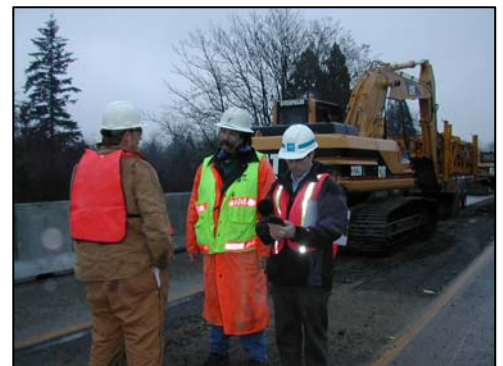
Construction Noise Measurement
