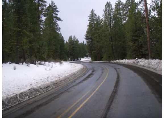
A narrow, icy roadway common in this section of OR 140.
