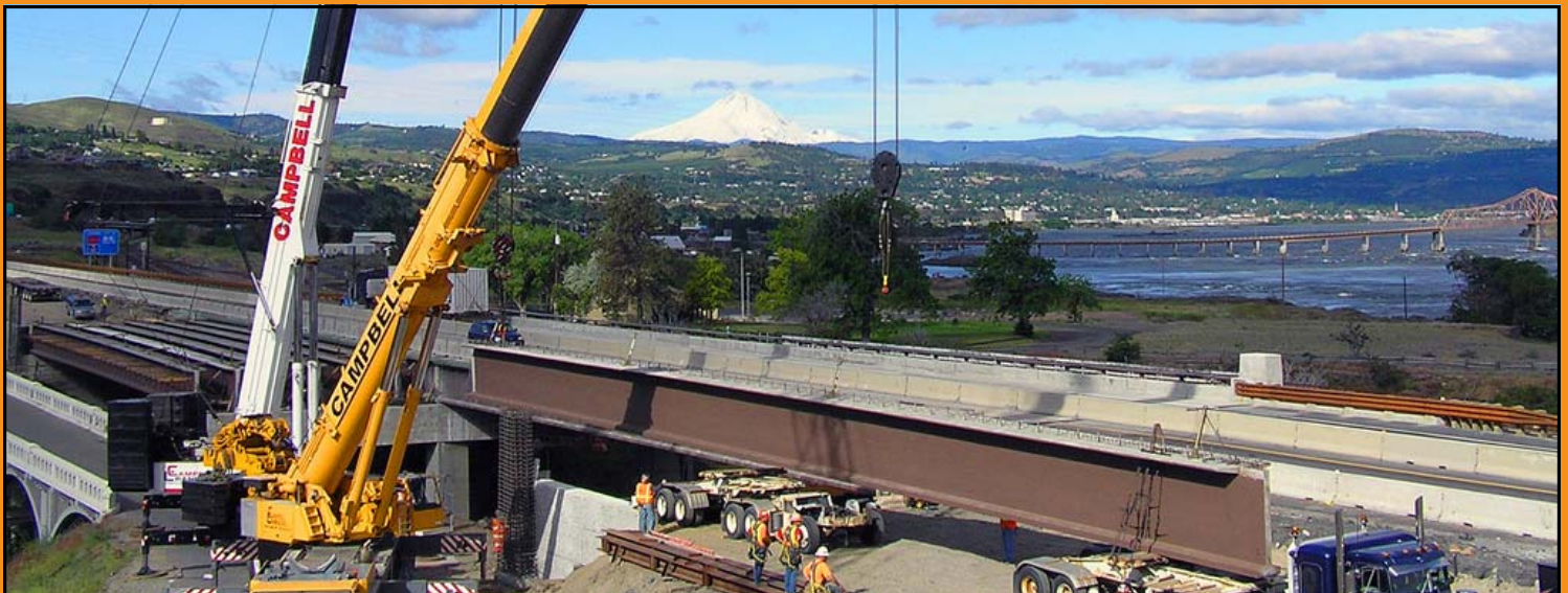
Beam swing operation on Interstate 84 at 15 Mile Creek in The Dalles, June, 2011. Beam swing operations can cause significant “gawking” or “rubbernecking” by passing motorists, which can reduce a work zone’s free flow threshold. (Background: Mount Hood; Right: Columbia River)
