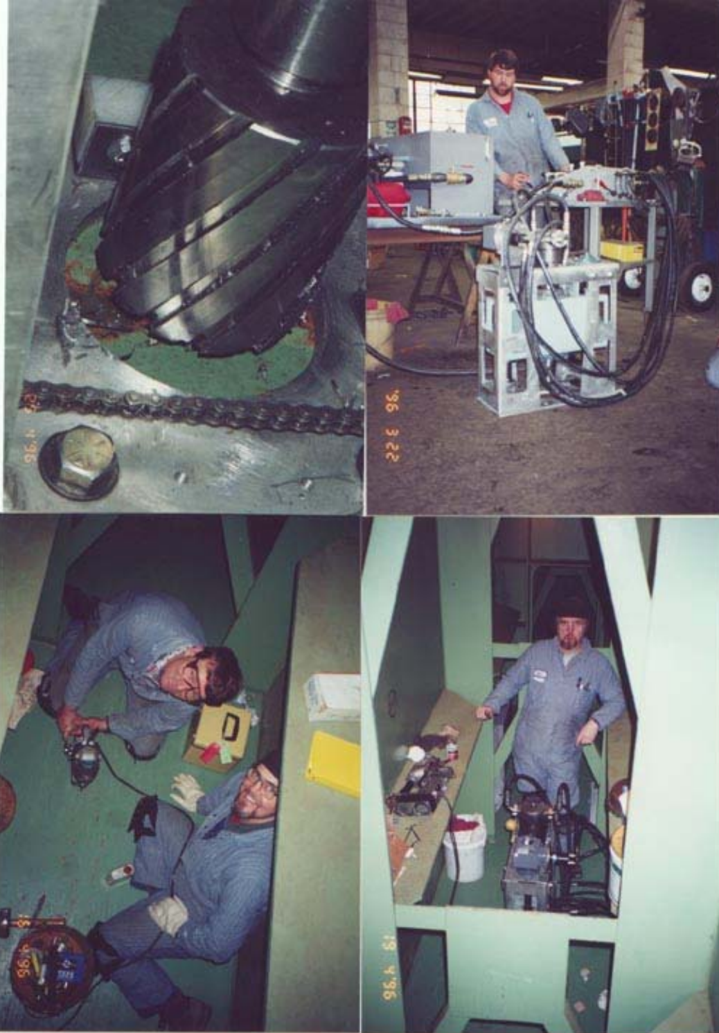
Figure 3.1: Coring ESW for material testing: 1) top left: close-up view of 4-inch diameter cutter; 2) top right: custom built drill; 3) bottom left: drilling and tapping mounting holes; 4) drill in place ready to core
