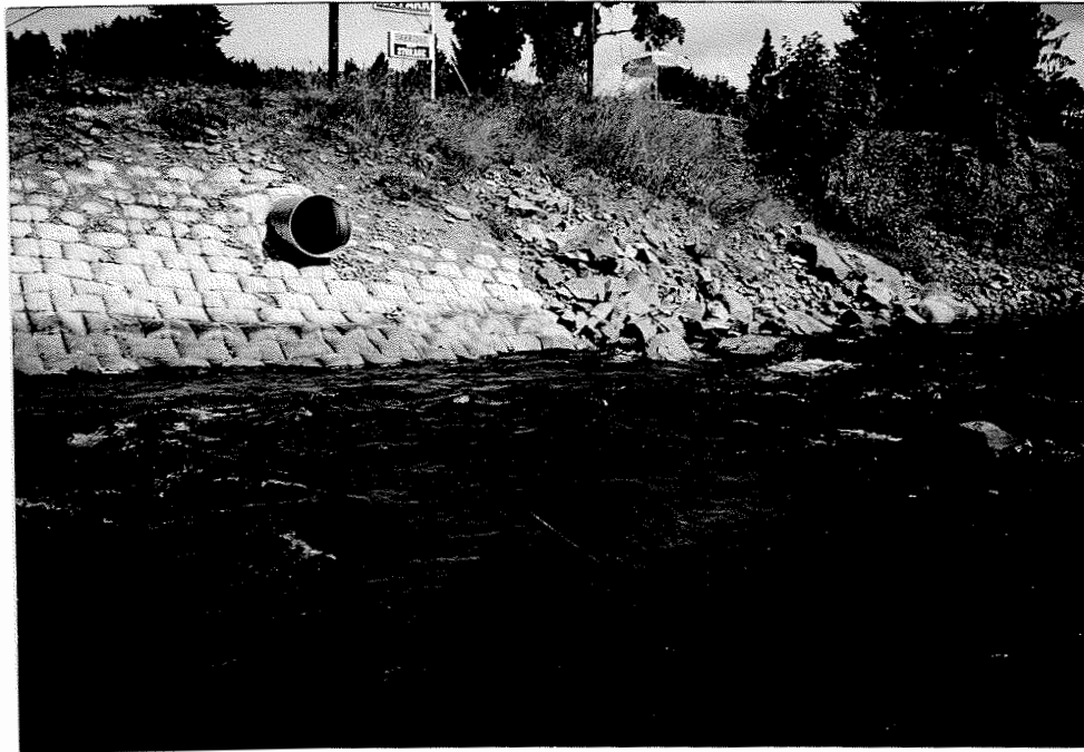
Figure 2.3: Northwest corner before flood, note the size of the riprap.
