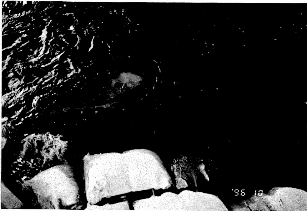
Figure 2.9: Exposed blocks after fill material in toe trench was scoured out.
