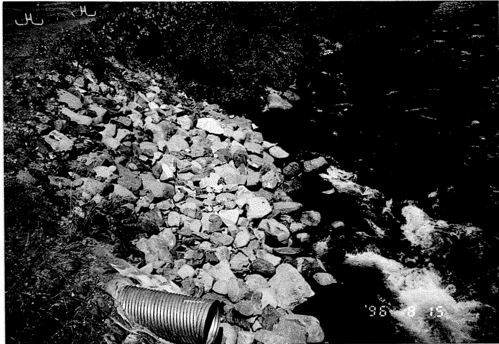
Figure 2.5: New riprap, note larger boulders in streambed near whitewater.
