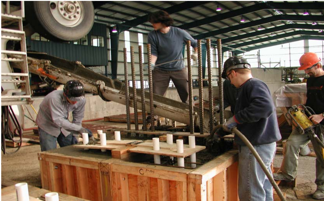
Figure 2.8: Placement of concrete into formwork
