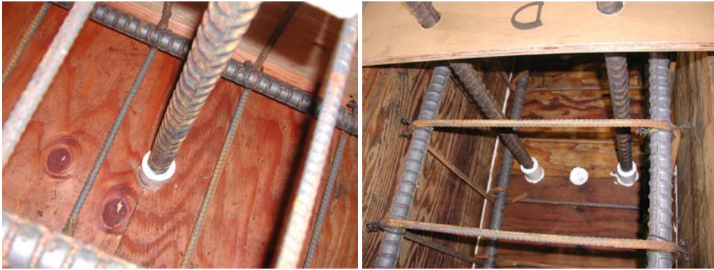
Figure 2.7: Typical PVC debonding pipe placed in specimens prior to casting
