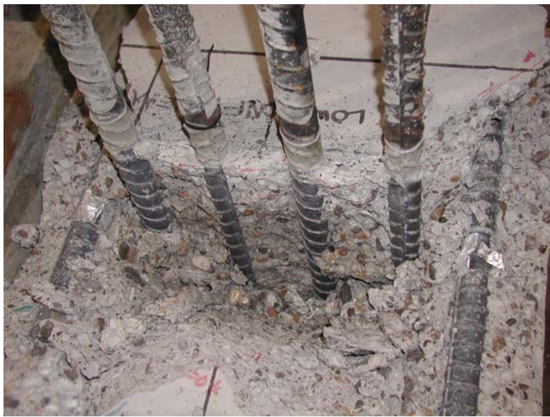
Figure 2.19: Visible concrete wedge penetration, concrete still in contact with reinforcing after failure
