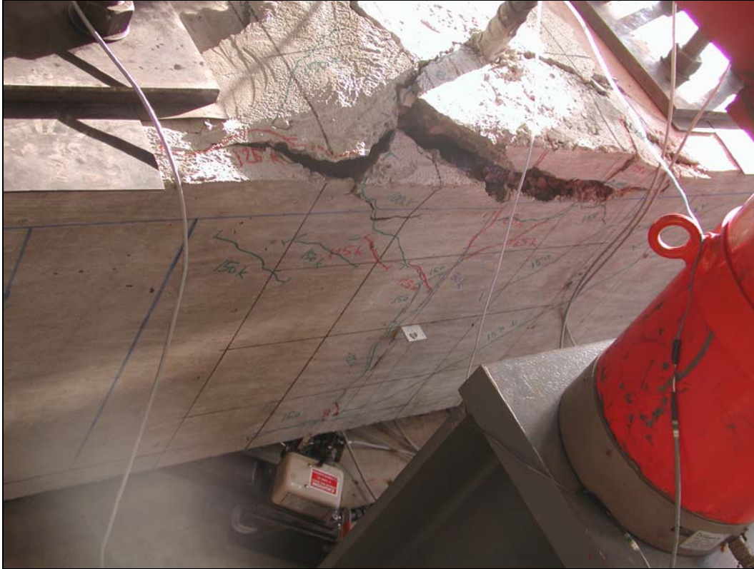
Figure 2.33: Specimen 2L0.21 at failure
