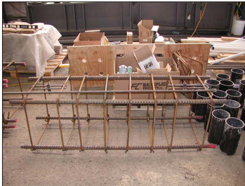
Figure 2.5: Typical medium confinement column cage prior to casting
