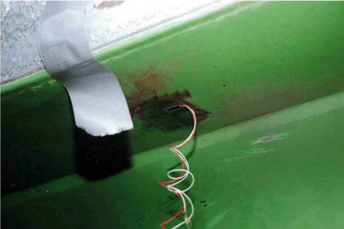
Figure 12 (71148-02) Strain Gage on Top Flange
