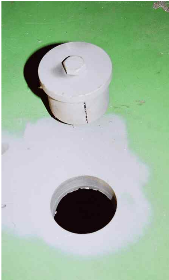
Figure 23 (71149-19) Core plug ready to be installed
