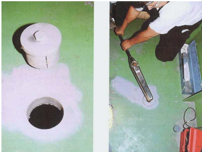
Figure 4.4: Core plug and core plug installation after core removal.
