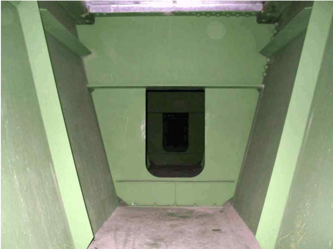
Figure 2 (D71055-19) Typical Appearance Inside of Girders
