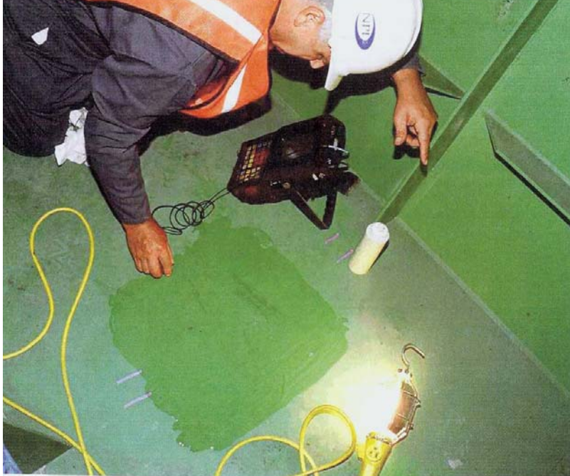
Figure 4.1: Ultrasonic testing of ESW prior to core removal.
