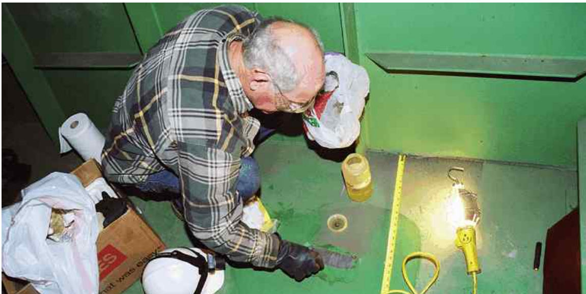
Figure 18 (71149-05) Weld being etched
