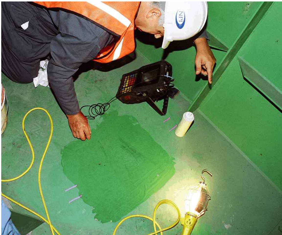
Figure 17 (71149-02) Ultrasonic inspection of weld prior to removing core
