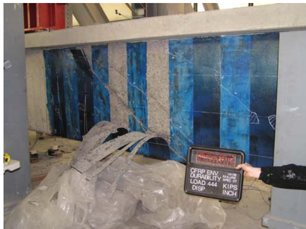
Figure 5.17: Failure photograph of Specimen T18Control
