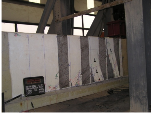
Figure 5.15: Failure photograph of Specimen IT12MCK
