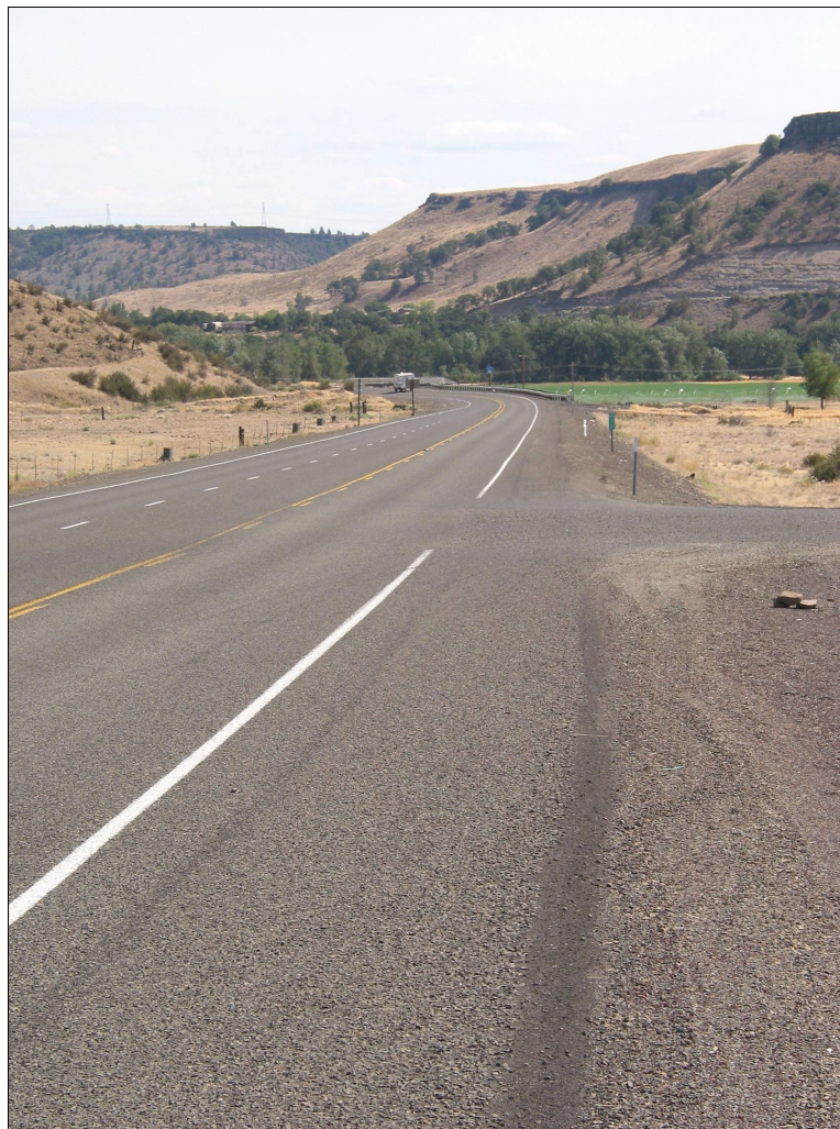
Figure 2.7: Photo of solvent-free (right) and solvent-loaded (left) sections after approximately 14 months
