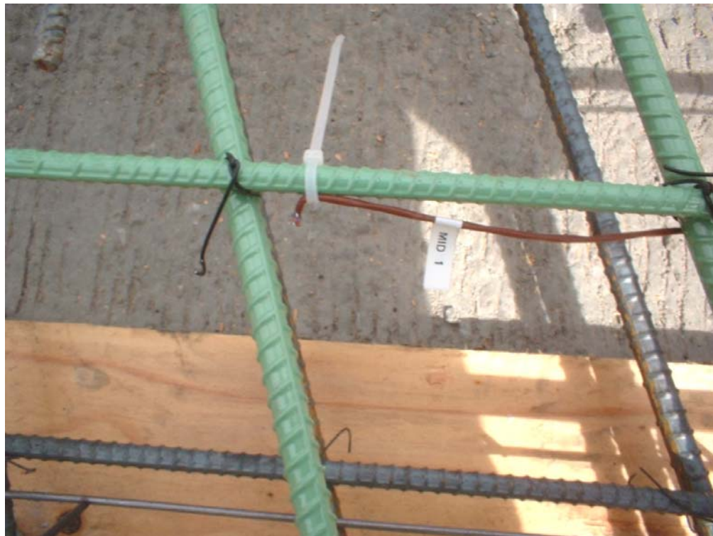
Figure 3.2: Attachment of thermocouples to the rebar
