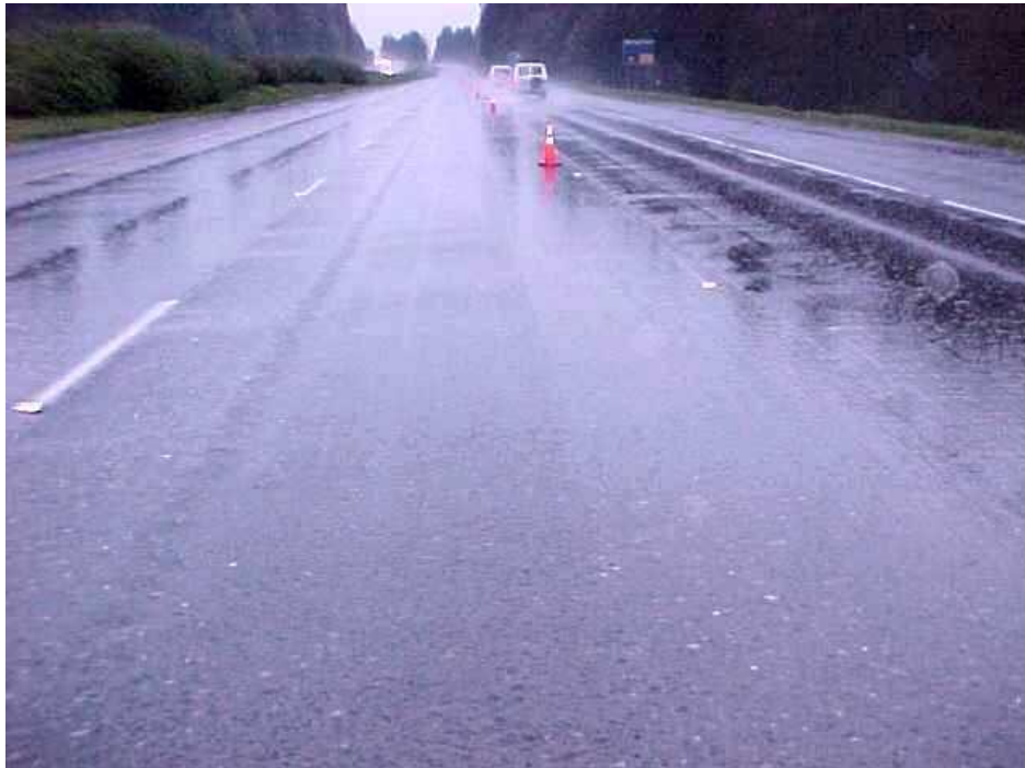
Figure 4.1: Post Construction Pavement Looking South (4/10/99)
