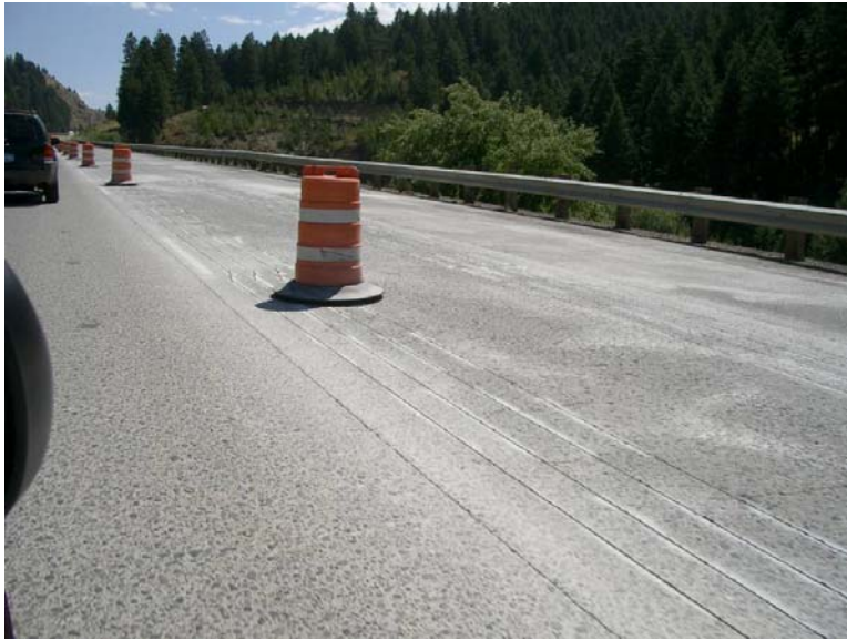
Figure 5.2: Pavement heating system under construction - I-84 near MP 271
