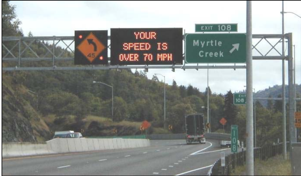
Figure 2.3: Example of a dynamic message sign for speed reduction, northbound, I-5, MP 108, Oregon
