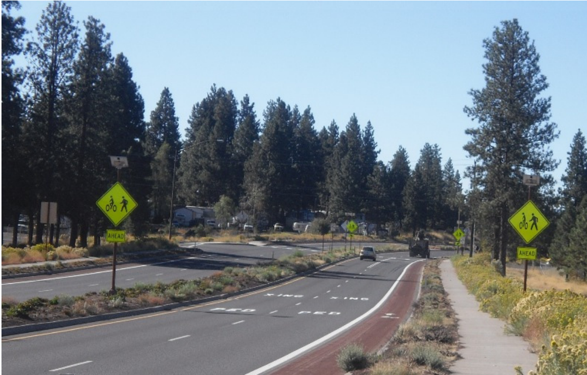
Figure 3.1 Driver's perspective of RRFB installation at the Bend Parkway and Reed Lane
