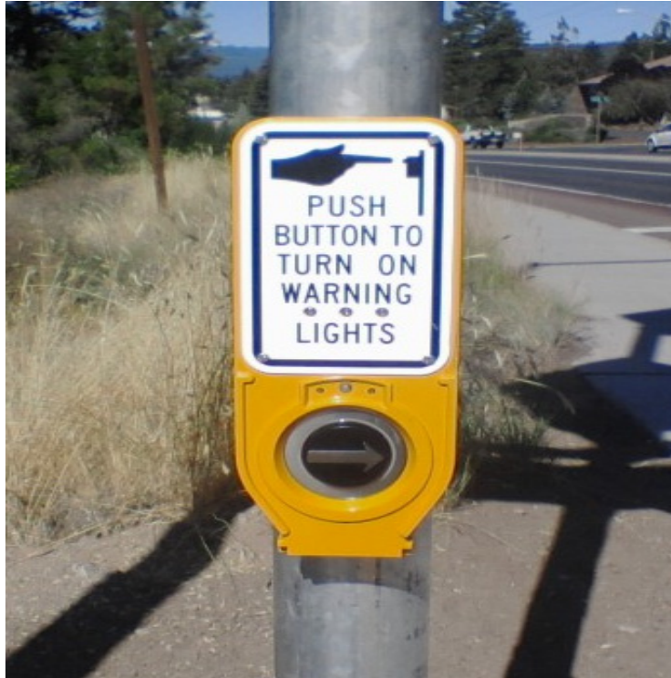
Figure 2.6: Pushbutton at Greenwood Avenue and NE 12 th Street RRFB location
