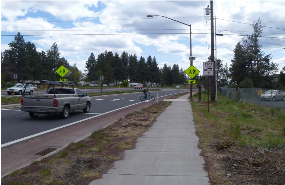
Figure 3.3: Bicycle crossing at the Bend Parkway and Reed Lane
