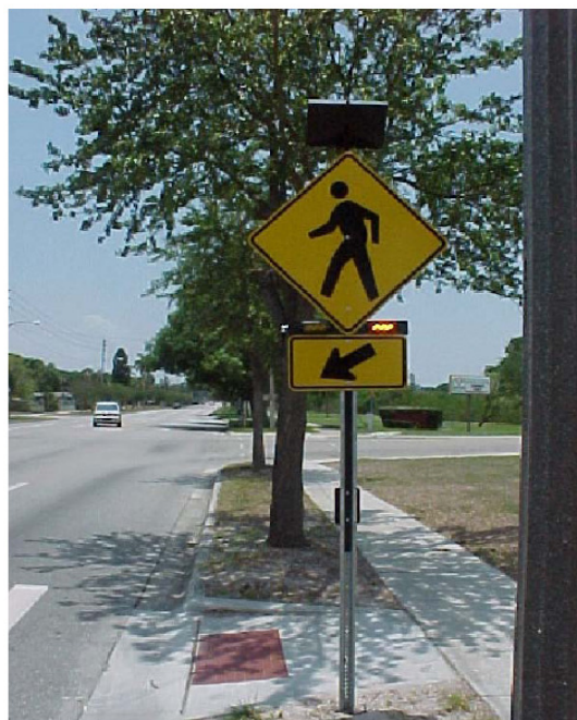
Figure 2.4: Rectangular Flashing Beacon Device (FHWA 2011)
