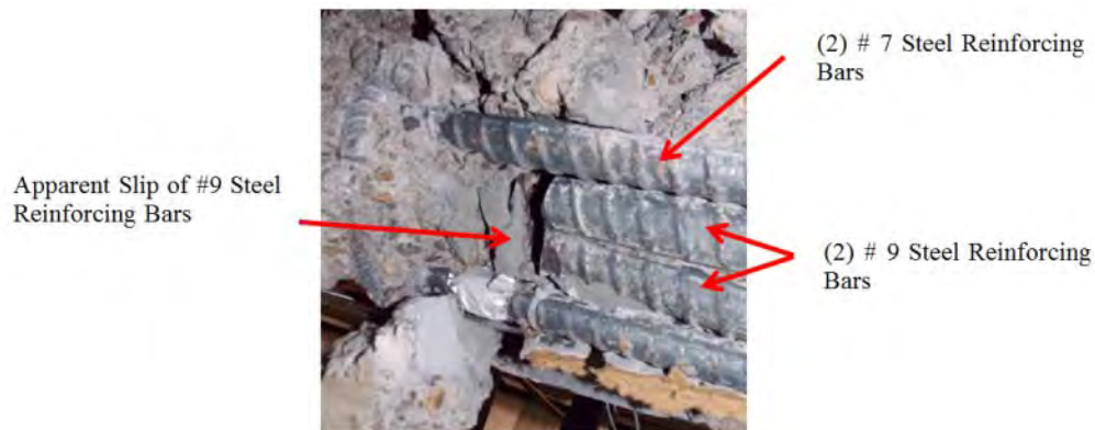
Figure D.27 - Apparent slip of # 9 Steel Reinforcing Bars in Mosier 2.
