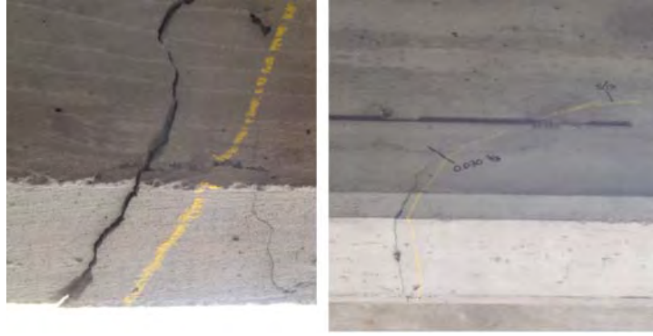
Figure D.3a – View of haunch transition on interior girder of span 1 (right) and crack with vertical offset on interior girder of span 1(left) (ODOT 2013)
