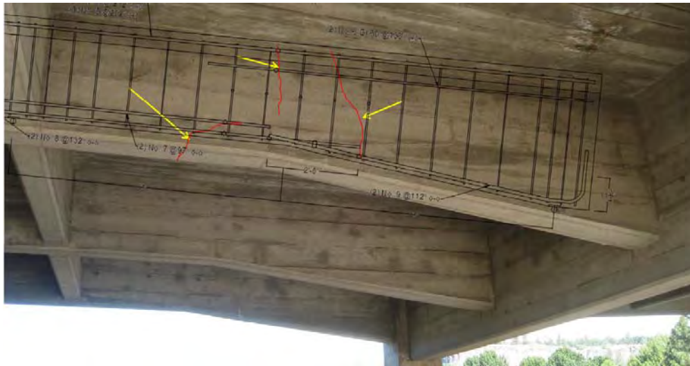
Figure D.3b – Overlay of reinforcing steel details on image of cracked girder.
