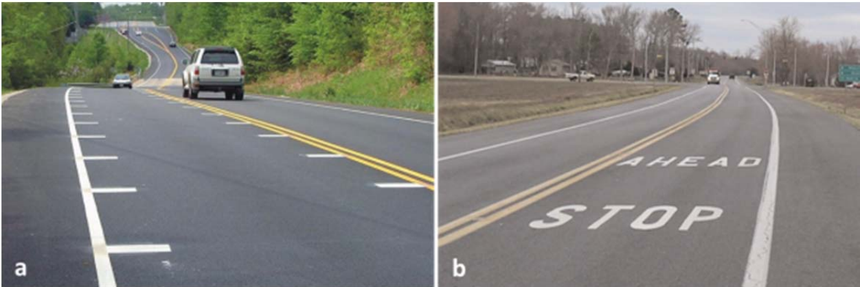
Figure 2.9: Example of Transverse Lane Markings and Warnings (a – (Arnold and Lantz 2007), b – (Gross et al. 2008))
