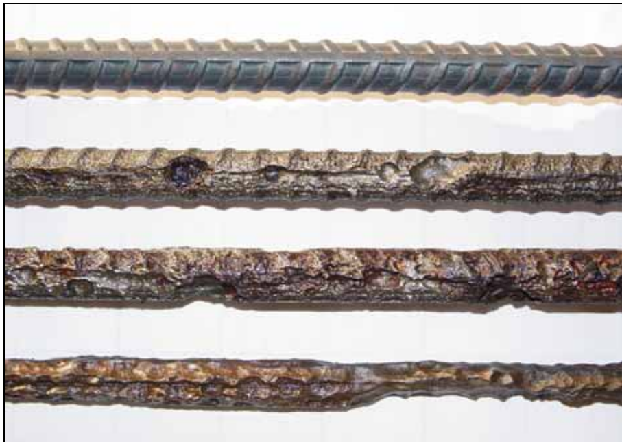
Figure 4.1: Different levels of corrosion on reinforcing steel removed from test beams (From top to bottom: A -Original, B - Light, C - Moderate, D - Severe)
