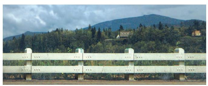
Figure 61—Two-Rail, Steel-Backed, Wooden Guardrail
