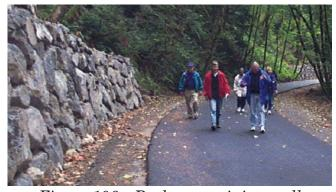
Figure 106—Rockery retaining wall
