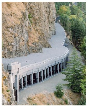
Figure 89—Rockfall Catchment from Above
