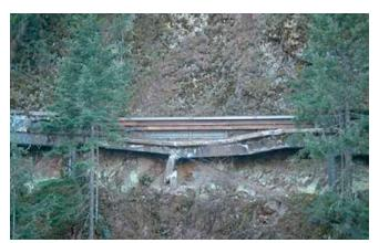
Figure 80—Damaged Eagle Creek Viaduct
