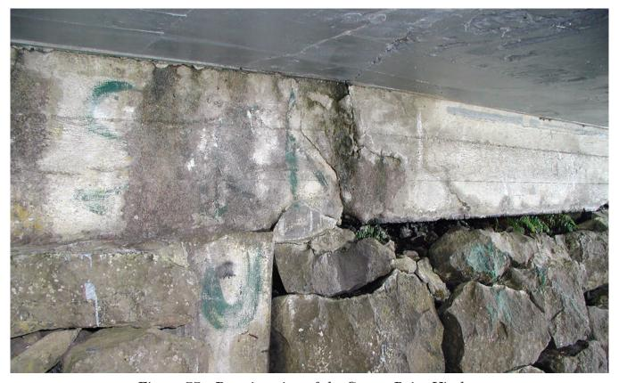
Figure 77—Deterioration of the Crown Point Viaduct
