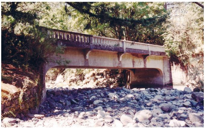
Figure 102—Tanner Creek Bridge Railing Repaired
