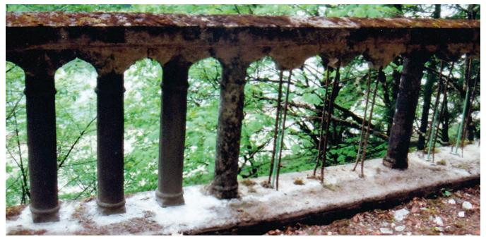
Figure 79—Toothrock Viaduct Railing deteriorated Condition
