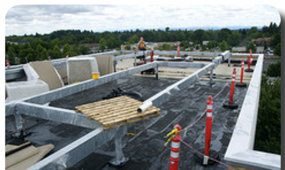
Frames for rooftop solar panels on T-Building.
