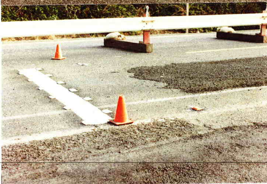
Details of northbound stop bar. Signal detector loop is under the pavement patch. Bar is of metallic tape.
