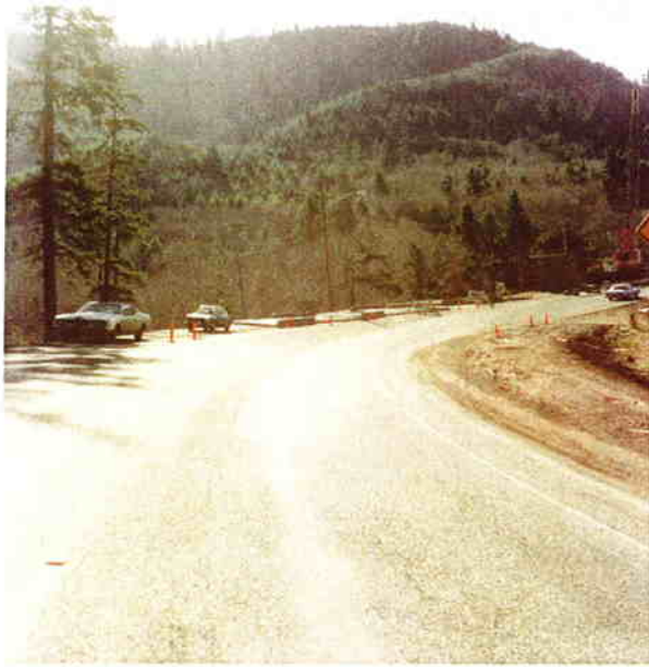
2/14/77 Looking south from 1869 at centerline reflectorized buttons on sunny day. Buttons barely visible.
