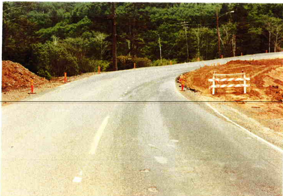
6/10/77 Southbound view from near sta. 1868.
