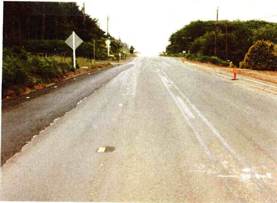
6/10/77 Southbound view from sta. 148. Raised markers and reflective tape are being used alternately.
