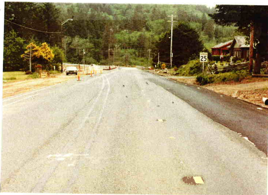
6/10/77 Northbound view from sta. 148. Note use of reflec- tive tape alternating with raised markers.
