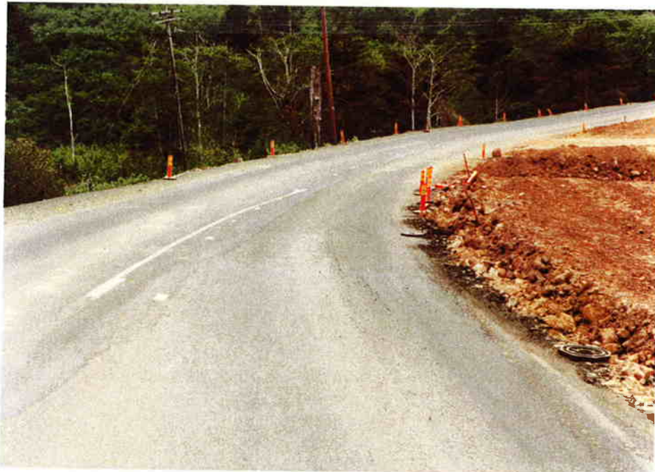
6/10/77 Southbound view from near sta. 1869.
