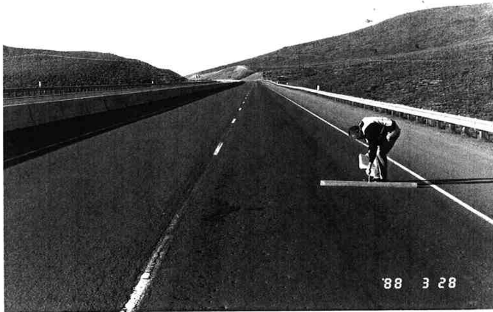
a) Milepost 305.8 Westbound
