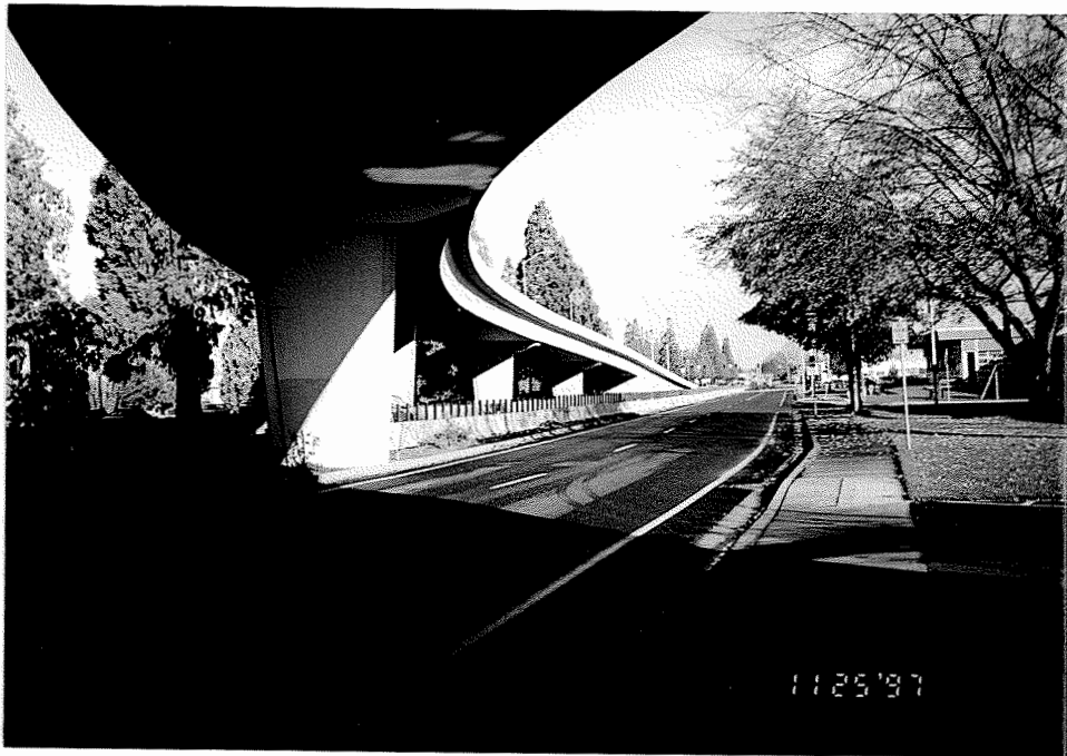
Figure 1.3 Bridge #9669A, wall-supported approach on the north end.
