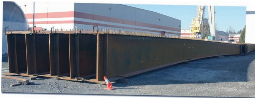
High-performance steel girders will support the Hilgard Interchange bridge.
