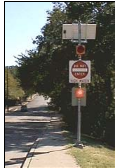
Flood Warning System Sign Assembly
