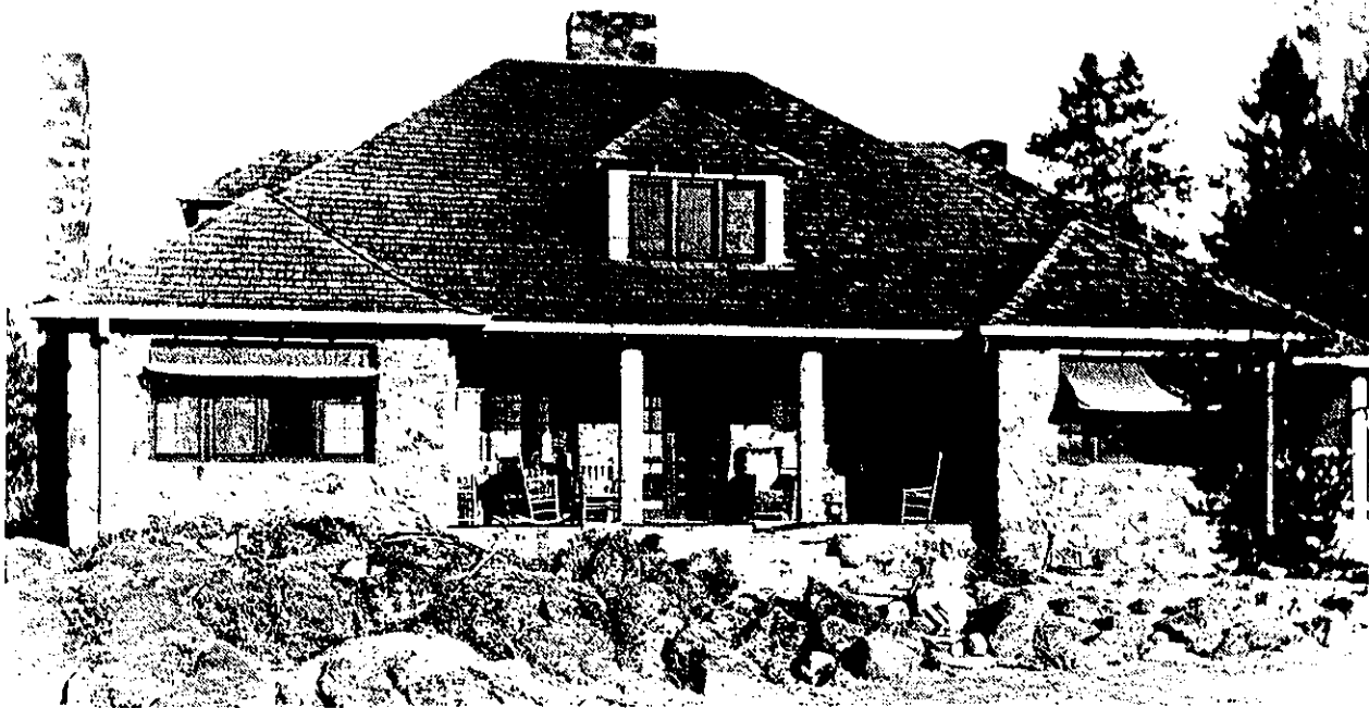
Fig. 3 Yamsi Ranch house at the end of construction in 1928 (OHS photo #55947.)
