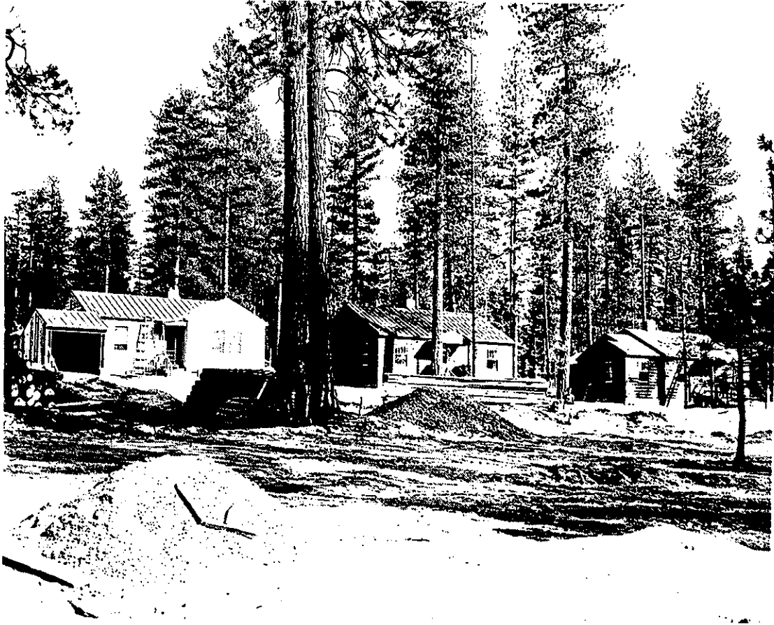
Fig. 4 Gilchrist houses under construction, 1940 (DHS photo #005678.)
