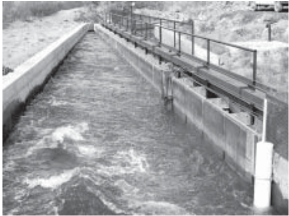
(Arnold Irrigation District diversion project with fish screens.)
