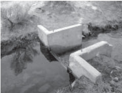
(Weir used to measure the quantity of flowing water.)
