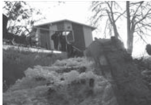
(Water is aerated before returning to Baker Creek)
