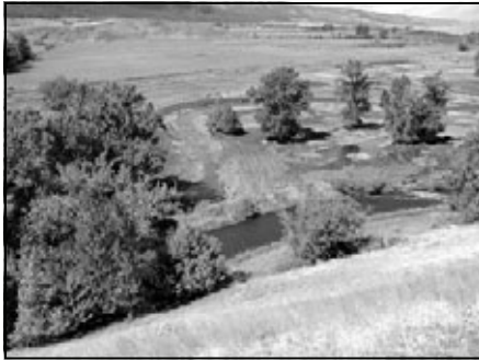
Early in the Wallowa River/McDaniel Restoration project, work proceeded behind the original channel, shown in the foreground. (left)
