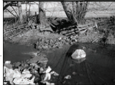
Fish-friendly rock weirs allow year-round fish movement through the entire reach of the Powder River.
