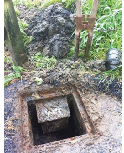
Cleaning out a catch basin at Coos Bay Yacht Club.
